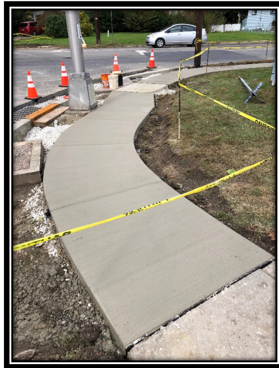
Figure 1: Contractor completed sidewalk at Somerdale Road.
