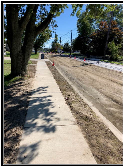
Figure 3: Recycled roadway surface ready for traffic.
