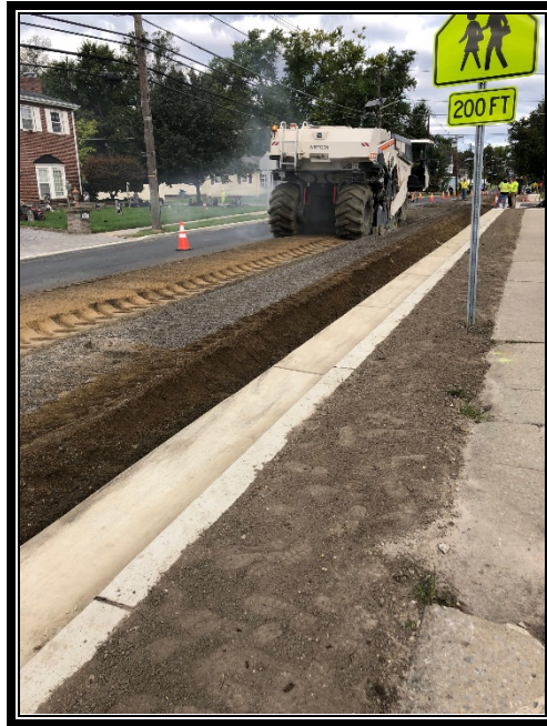
Figure 2: Contractor performing roadway recycling between Wood and Earl Avenue.
