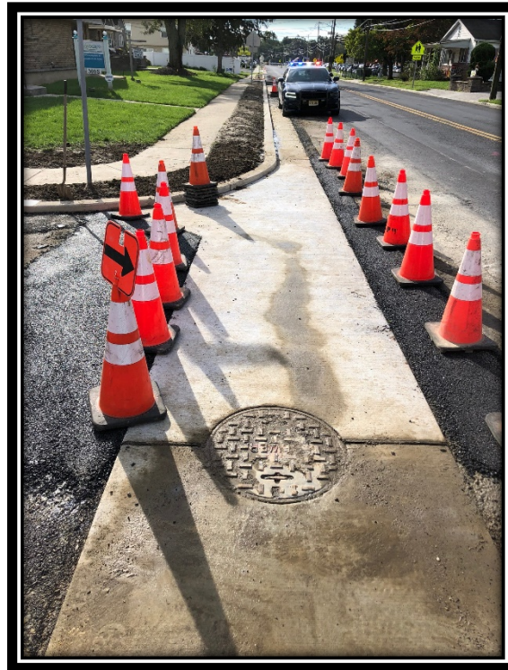
Figure 1: Completed slope gutter at Wood Avenue.
