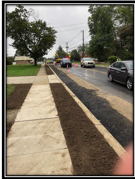
Figure 1: New sidewalk and curb with restoration near Wood Avenue.
