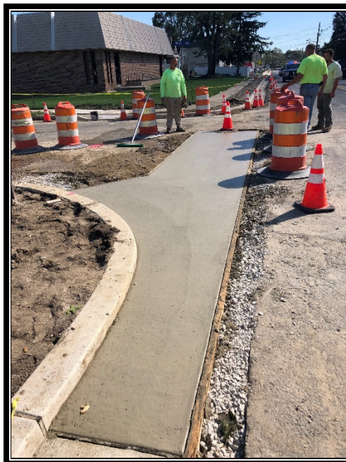
Figure 3: Installing slope gutter at Wood Avenue.
