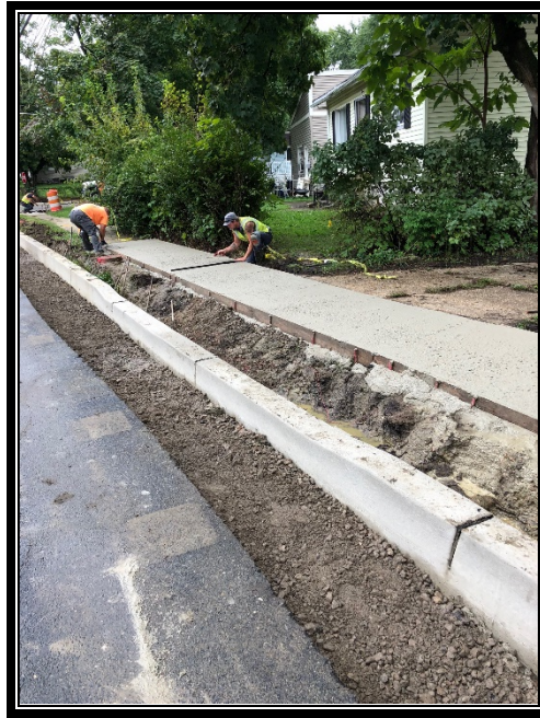
Figure 2: Completed curb and sidewalk on the west side of Warwick Road.
