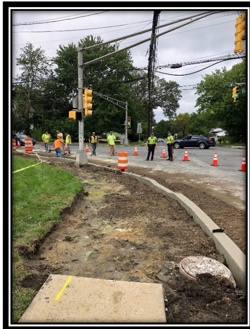
Figure 1: New curb at Somerdale Road..
