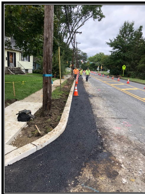
Figure 3: Restored area at Earl Avenue.
