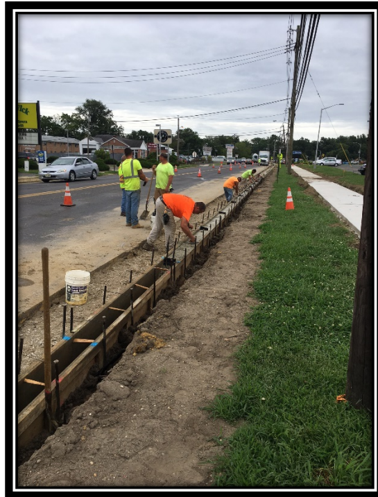
Figure 1: New curb in front of Sterling Highschool.
