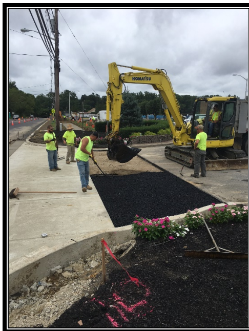
Figure 3: Asphalt pavement tie into parking lot at Sterling Highschool Main driveway.
