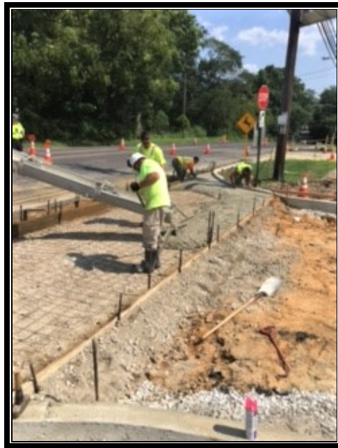
Figure 2: Concrete Driveway, 6" Thick at Sterling Highschool.
