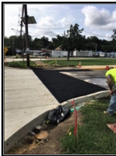
Figure 3: Asphalt pavement tie into parking lot at Sterling Highschool south driveway.
