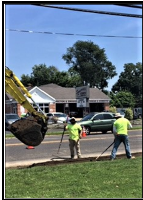
Figure 3: Backfilled area in front of Highschool where sidewalk was removed.
