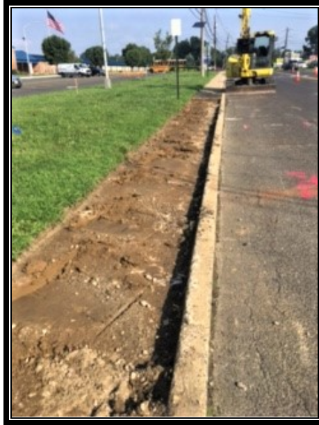
Figure 2: Removing sidewalk at Sterling Highschool.
