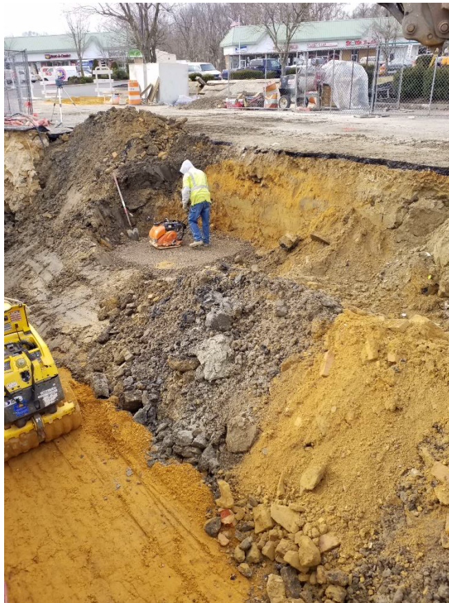
Contractor preparing the area where an inlet will be placed
