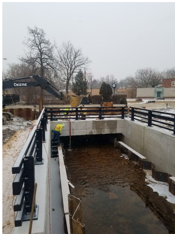
Railing on both wingwalls and on culvert
