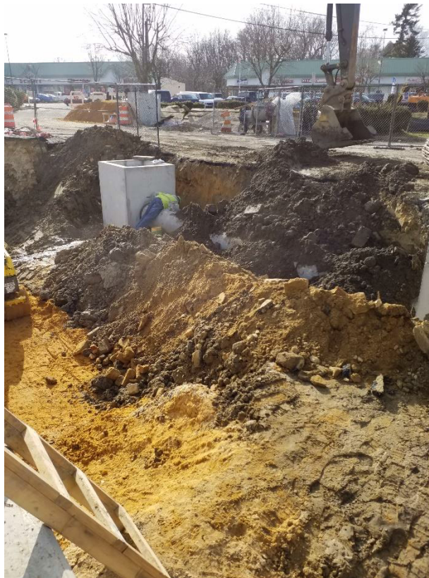
Inlet placed, and drainage pipe connected to the inlet in roadway
