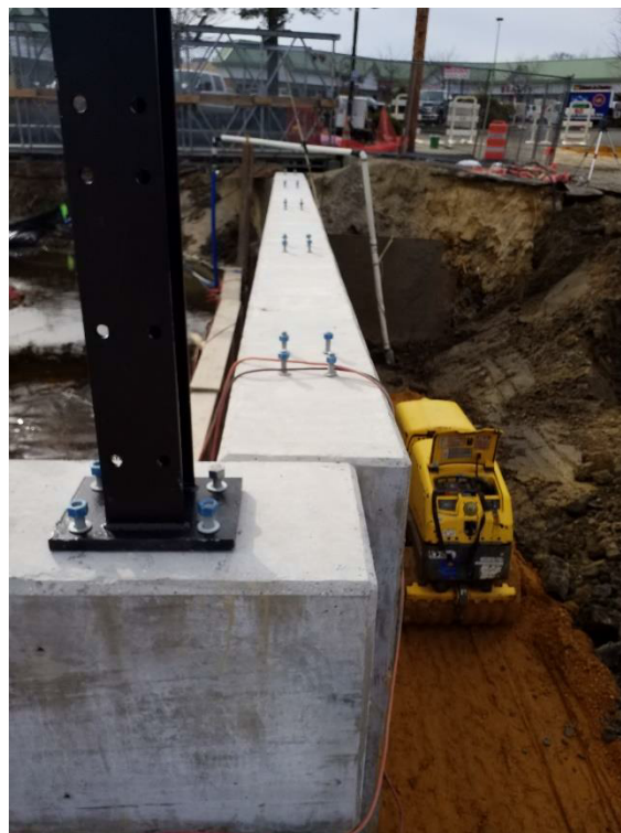
Bridge railing is being placed
