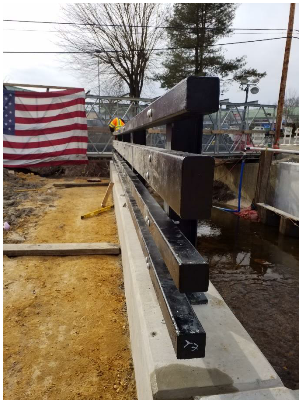
Railing on the wingwall
