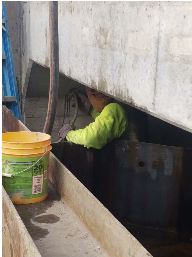
Contractor using grout pump to install grout in the tube for the post tensioning strand
