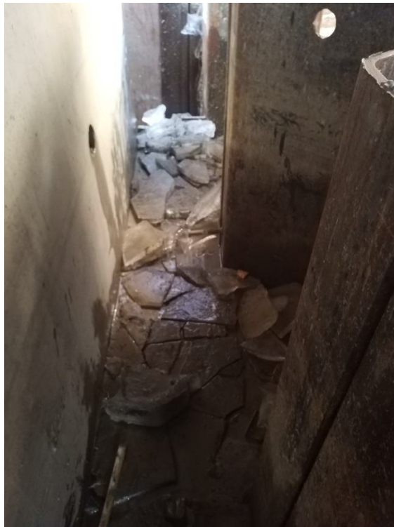
Area between sheets and culvert had water laying which froze in the cold temperature
