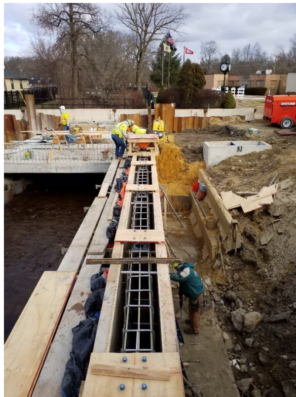
Forms all set and anchor bolts in place for railing
