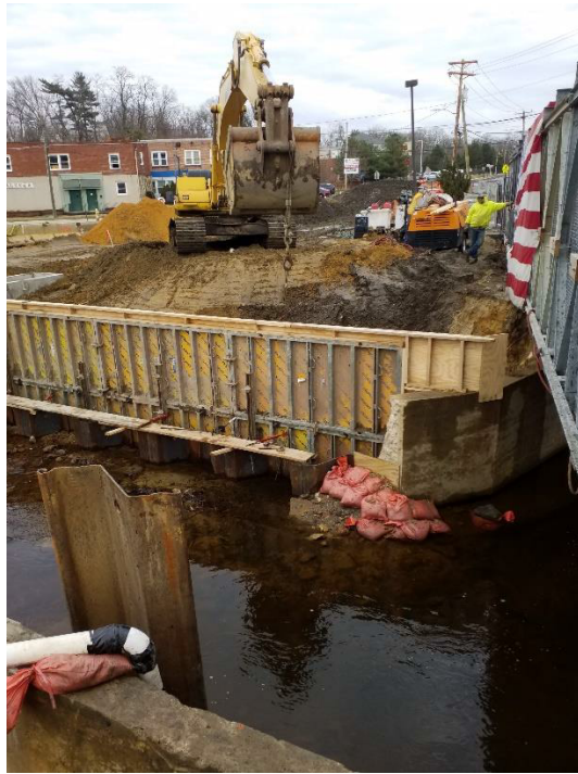
East side wingwall forms looking at it from the west side
