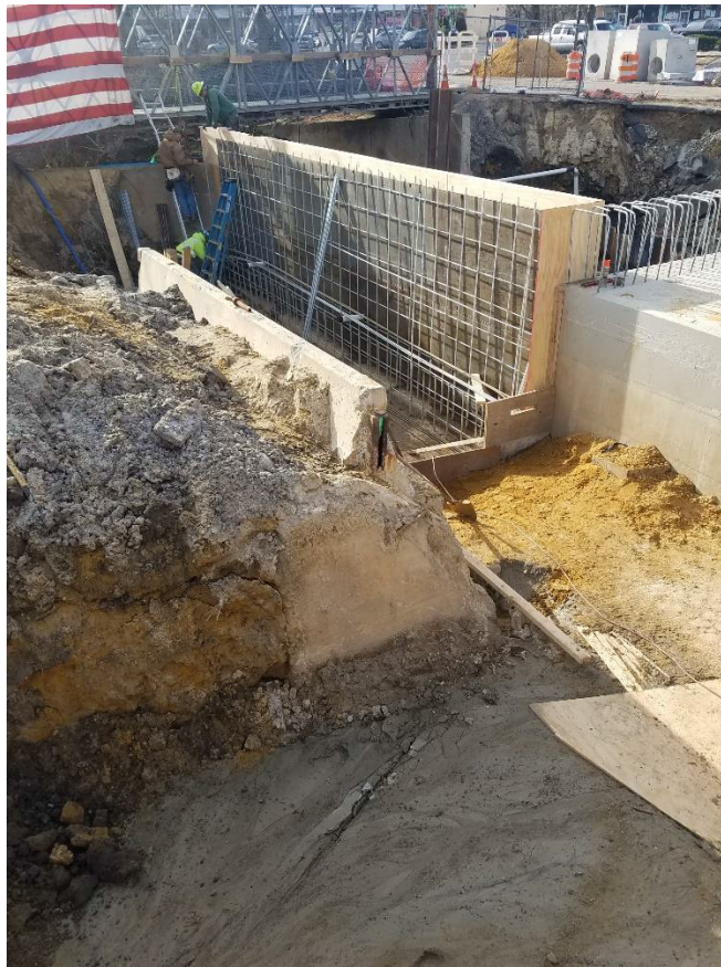
Installed re-bar and setting forms for Wingwall on East side
