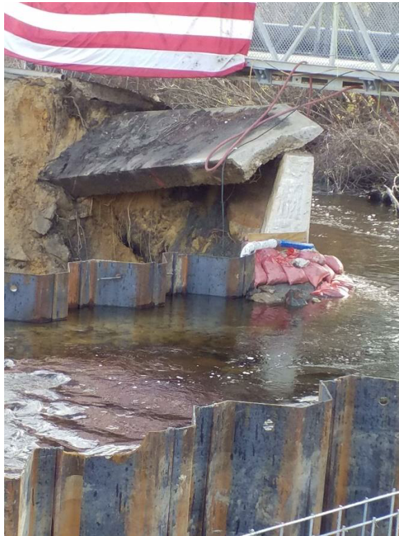
Existing slab was undermined due to rain. Slab was removed
