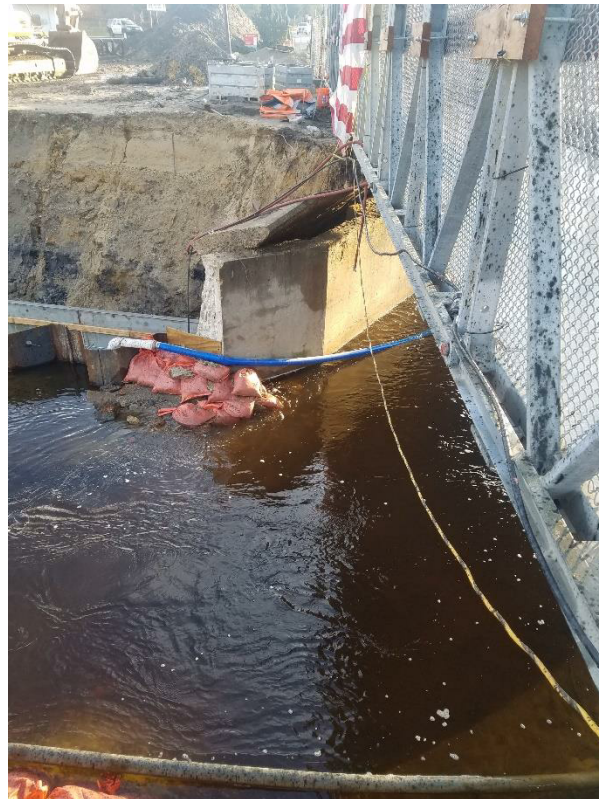
More sand bags needed to be placed to keep water out
