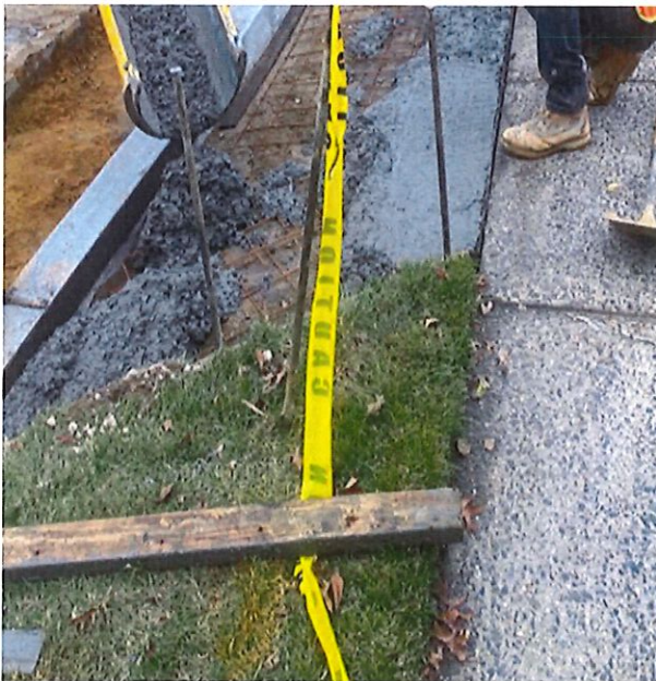
Figure 4: Concrete apron placement
