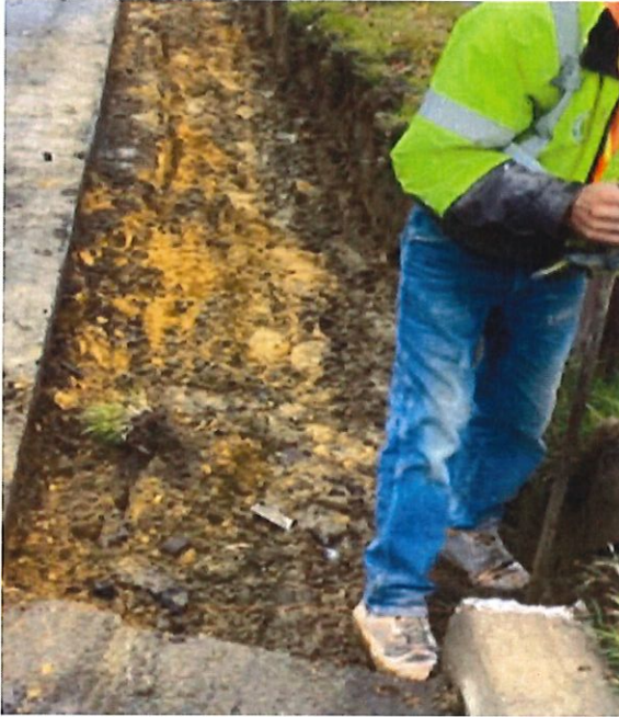
Figure 2: Removal of asphalt, curb, and aprons
