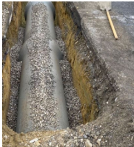
Figure 1: Pipe with stone base
