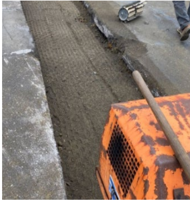
Figure 2: Compacting DGA
