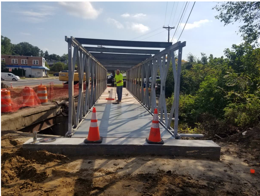
Not skid surface being installed
