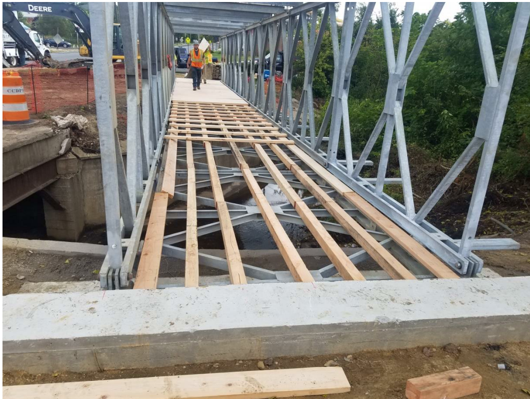
Pedestrian bridge was erected and flooring is being installed
